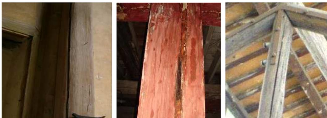
Figure 1: Longitudinal cracks in historical timber structures
