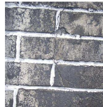
*Figure 2: Crack on top of brick arch Broken top of brick lintel arch Vertical crack in the joint of walls*
