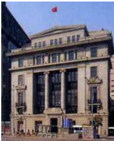
Figure 4: Picture of the Bund 18 building
