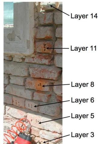
*Figure 2: Position of micro-cores samples in the brick wall of the monastery*
