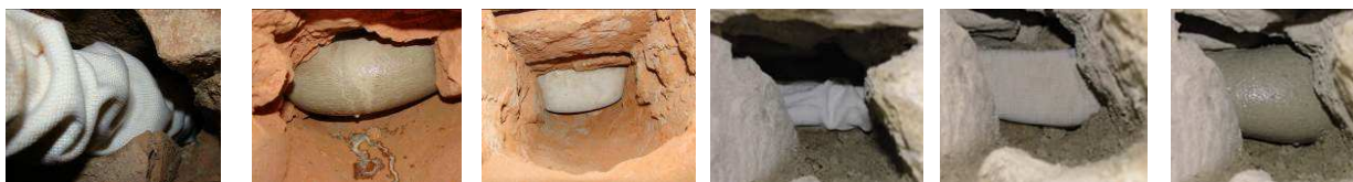
Figure 1: Injection phases into brick masonry and stone masonry
