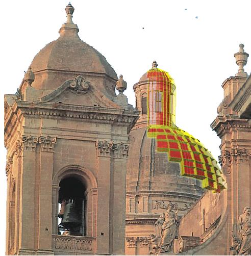
Figure 2: Macro-element meshing of a dome
