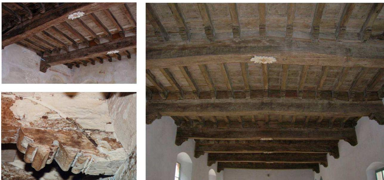
*Figure 3: The wooden floor before restoration*
