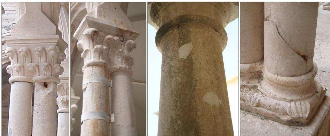
Figure 1: Column connection with specific fractures
