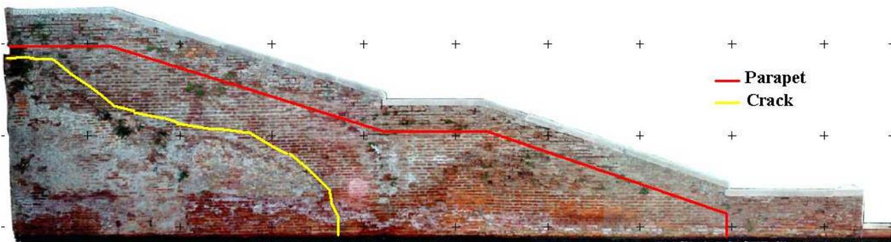
Figure 17: Main crack on North side of the central staircase
