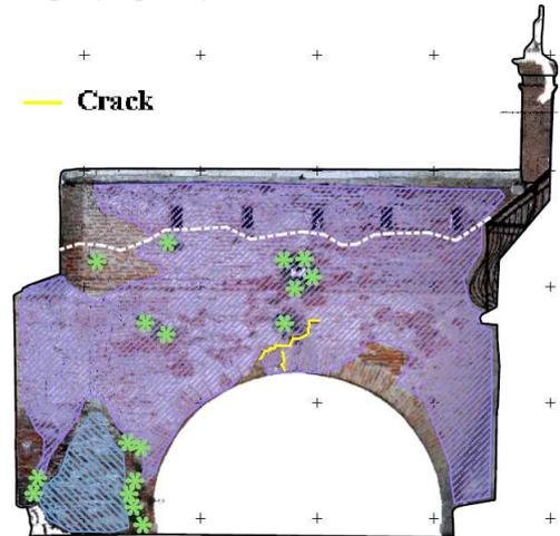
Figure 13: Cracks on the North side of the bridge
