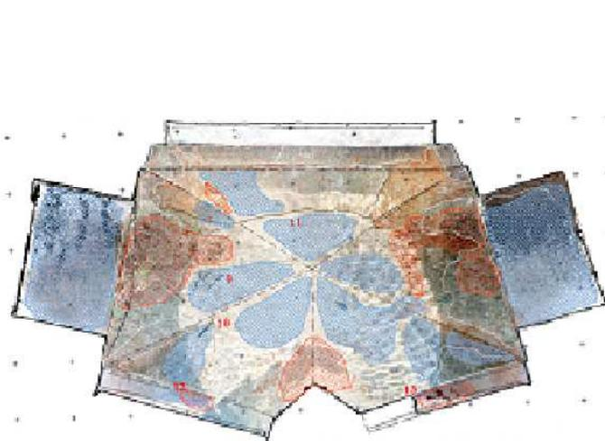
Figure 3: Relief laser scan of the vault
