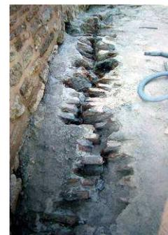
Figure 11: Cracks on the cross vaults of gallery, 2001
