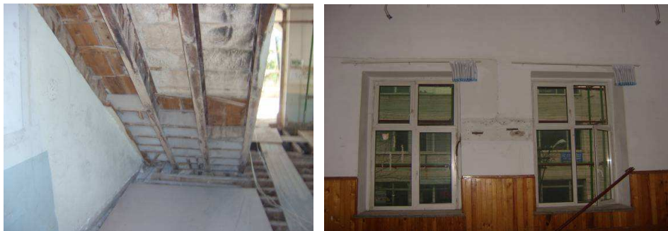
Figure 7: Existing situation of stairs and windows
