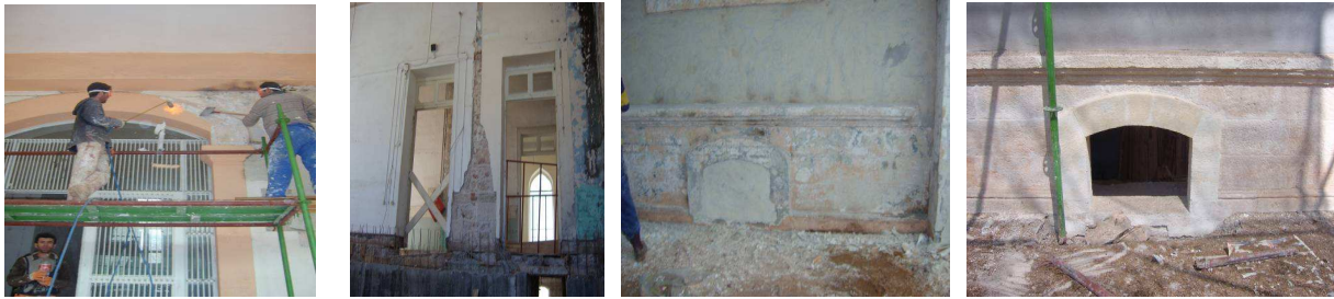
Figure 9: Picking up grouts and paints
