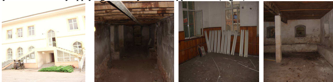
Figure 3: Picture of existing situation of structure
