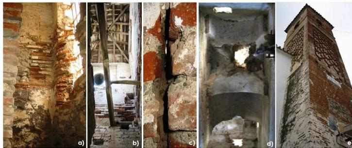
*Figure 1: most significant damages and general view (a) view of the NE-NW inside corner and the core: spalling and loss of material; (b) wooden roof detail; (c) passing-through crack at southwestern wall; (d) perforated vault; (e) north-eastern and north-western façades*
