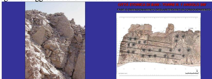
*Figure 5: View of the damage in the tower and drilling plan, which includes orthogonal and slanting drillings for glass fiber reinforcements, Citadel of Bam, Iran. (Credits: Engineer. Valter Santoro, 2008)*
