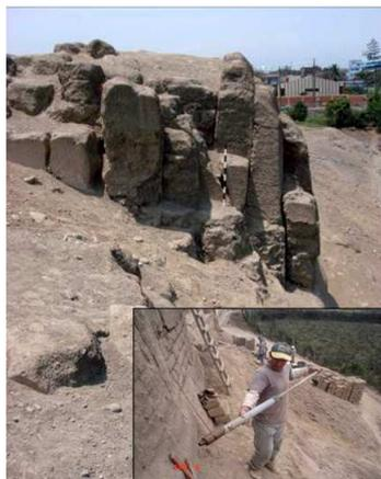
*Figure 3: Weakened containment wall, injected with mud grouts to increase its strength to side filling tension (Credits: Mirna Soto, 2008)*
