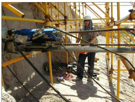
*Figure 6: Scaffolding, drilling and placement of glass fiber rods. Bam Citadel, Iran
