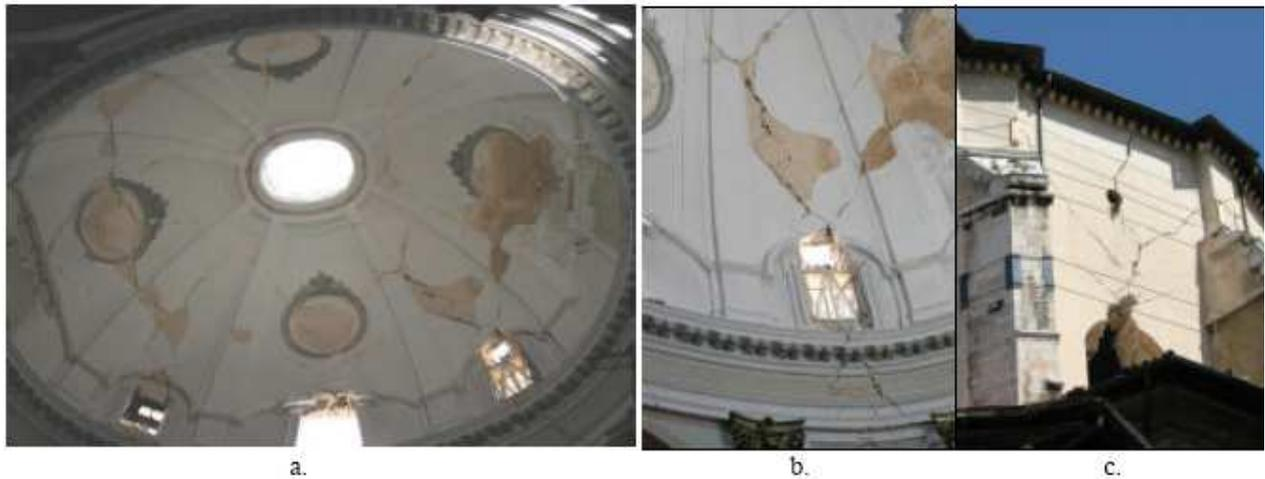
*Figure 6: Crack in the dome and in the dome cladding*
