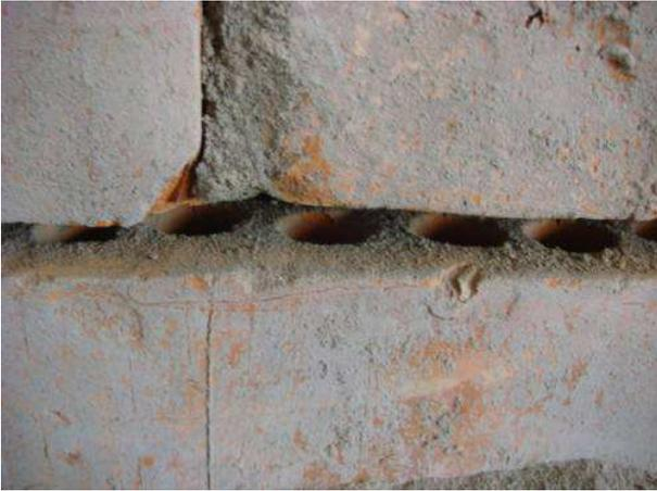
*Figure 3: The wall before mortar replacement (no mortar in the brick holes)*
