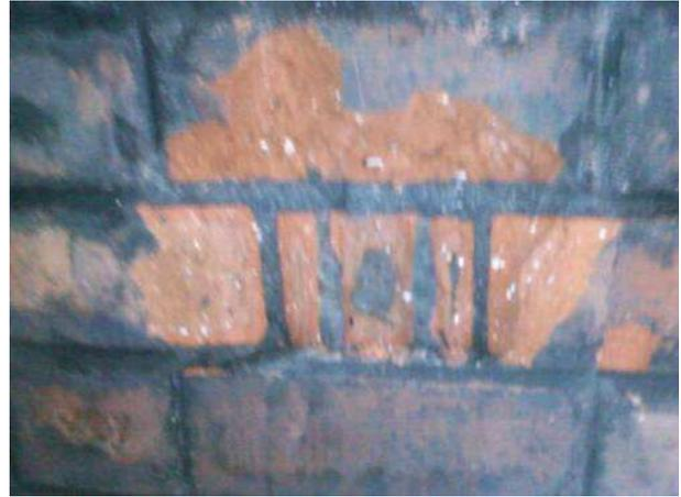
*Figure 4: The wall after mortar replacement (brick holes is full of mortar)*
