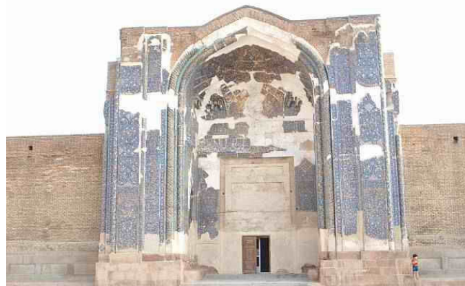
(b) Kaboud Mosque of Tabriz Damaged by the Tabriz earthquake (1721)
