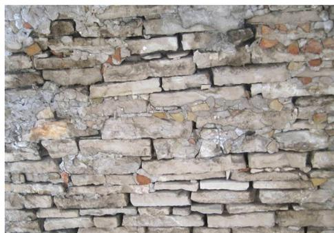
**Fig. 3** Degradation process on intrados
