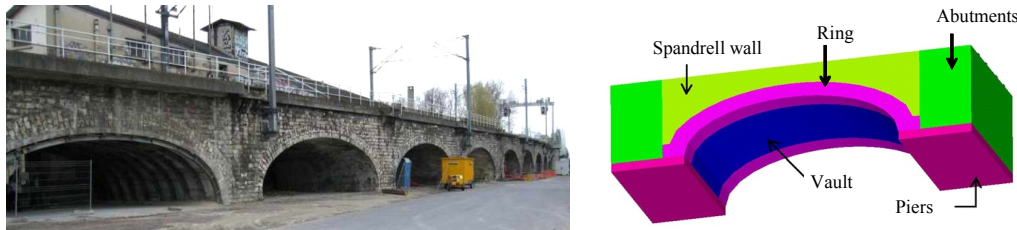
Fig. 2 The masonry bridge studied (9 spans about 12.50 m long, 8 m wide). Archive plan 1904
