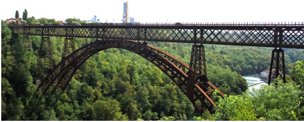
Fig. 1 Present up-stream view of the iron arch bridge (1889) from Paderno d'Adda (right bank)
