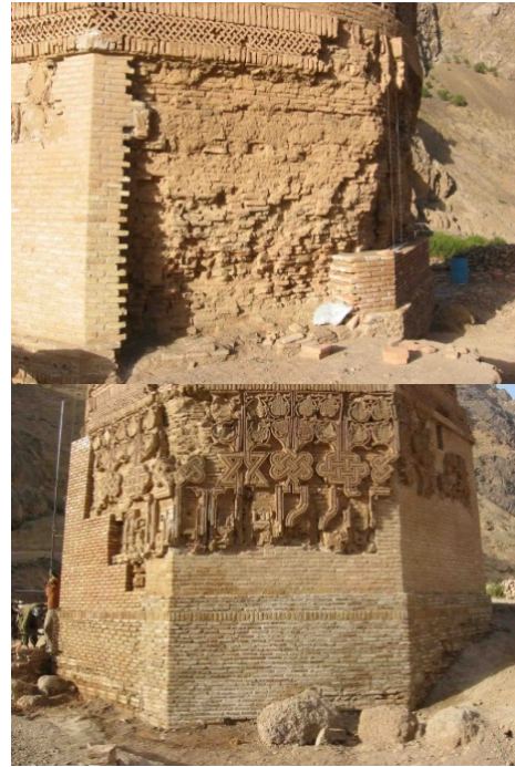
Fig. 2 Consolidation works at the basement
