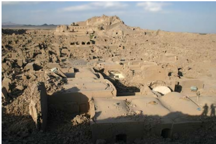
Fig. 2 Arch net, Digital library, Citadel of Bam, general view, post-earthquake
