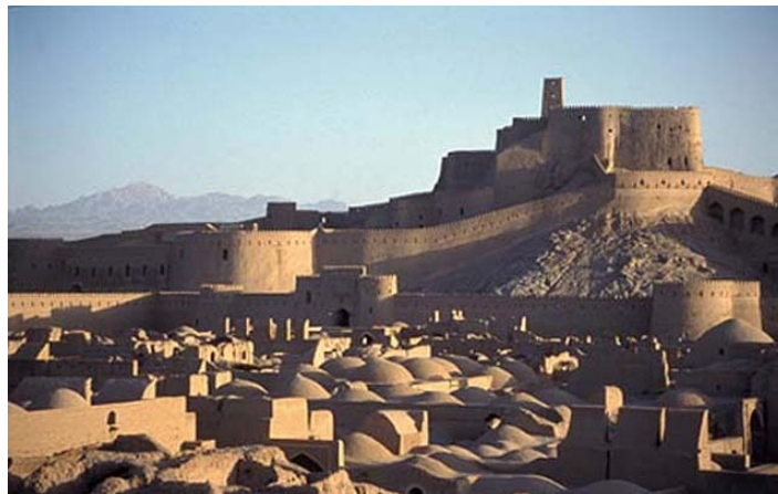
Fig. 1 Arch net, Digital Library, Citadel of Bam, general view, prior to the earthquake.
