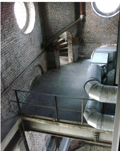
**Fig. 3** Access to the roof is limited by the ventilation system
