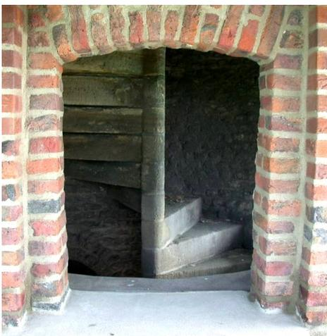
Fig. 5 Reactivated fire escape stairway
