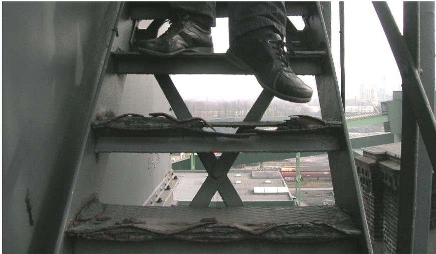
**Fig. 2** The shaft tower is standing inside an active mining plant, stairs are destroyed beyond repair
