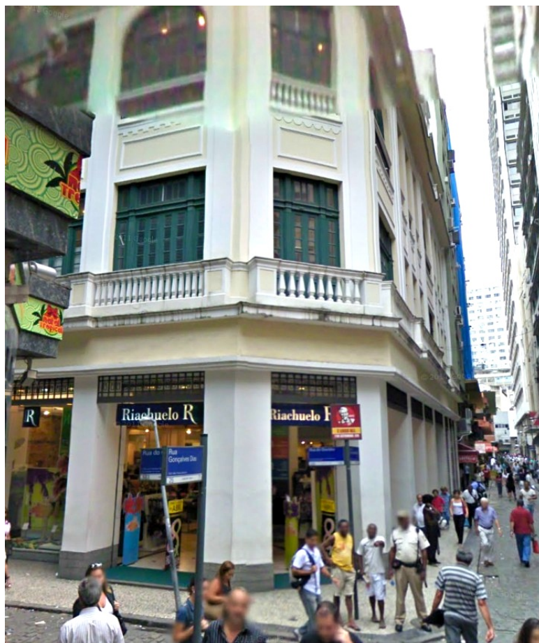
Fig. 2 Example of inappropriate use in relation to the building’s typological vocation: located at Rua do Ouvidor, 158-162, within the Cultural Corridor protection area
