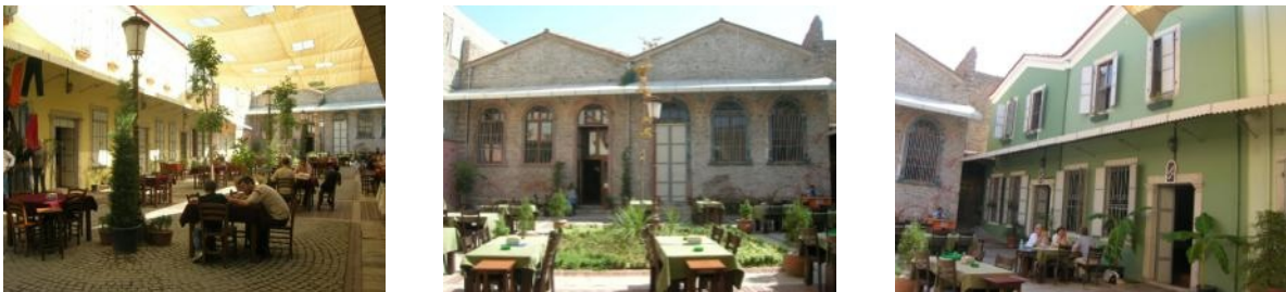
Fig. 19-21 Abacioglu Han After Adaptive re-use Attempt (Mine Tanac Zeren Archive)
