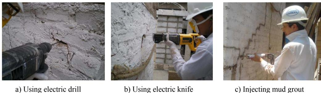
Figure 5. Opening seismic cracks and injecting mud grout.
