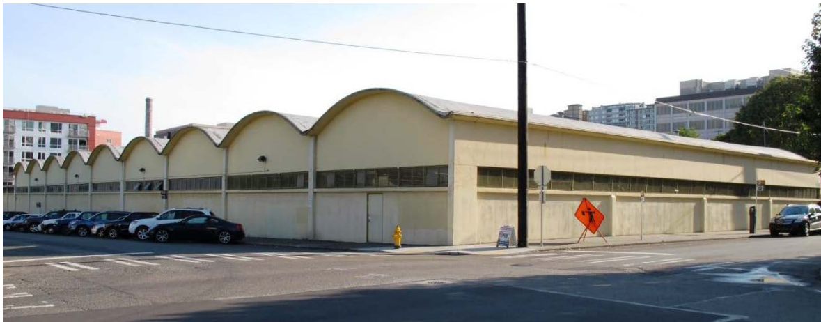
Figure 1. Seattle School District Warehouse
