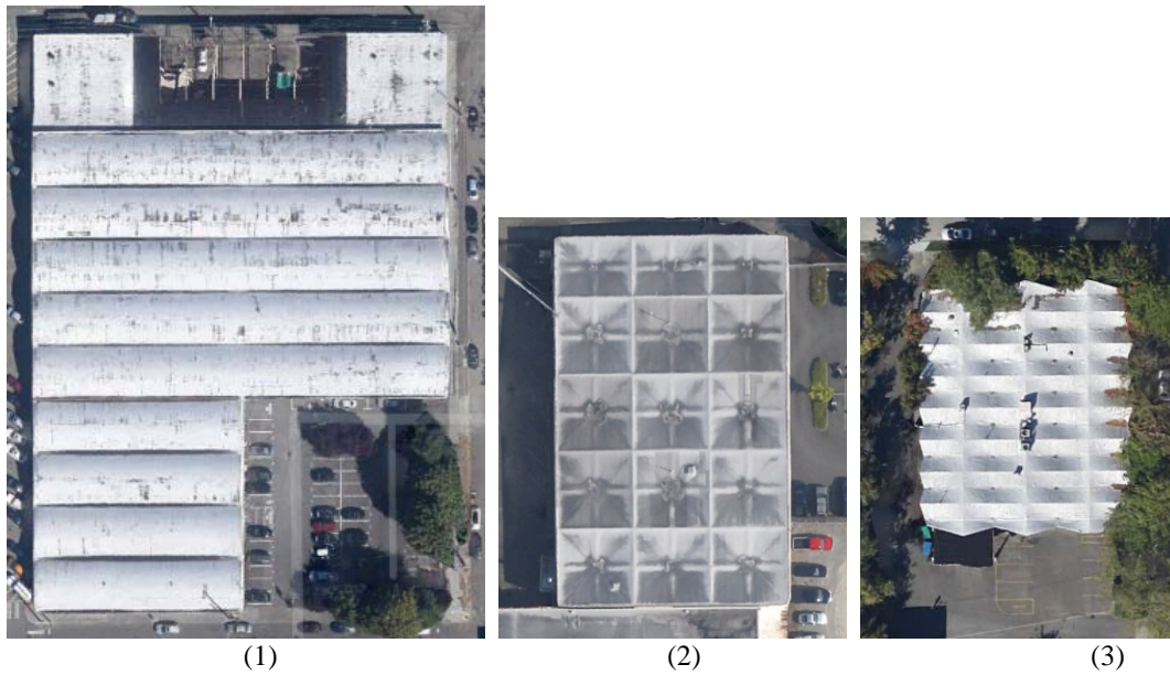
Figure 2. Aerial View of Barrel-vaulted warehouse (1), hyperbolic paraboloid umbrella warehouse (2), and gabled hyperbolic paraboloid office building (3). (Not to scale)
