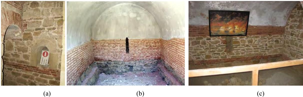
Figure 6: Powder magazines of Namazgah Bastion, (a) brick arche and niche 2013, (b) vault and brick walls which were placed on rubble stone foundation walls, 2007, (c) brick and rubble stone alternating wall and ventilation holes, 2013.
