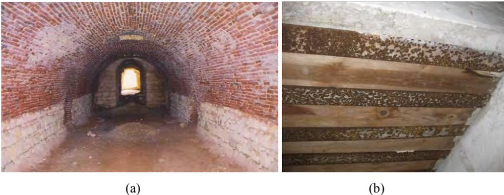
Figure 8: (a) brick vault on masonry foundation walls of garrison and quarter of Kırklareli Seyfioglu Bastion, 2004, (b) reinforced concrete slab supported by steel profiles of Canakkale Anatolia Mesudiye Blockhouse, 2013
