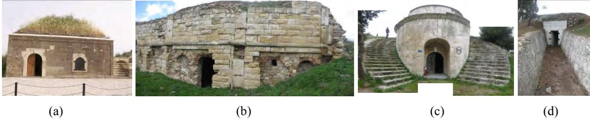
Figure 7: (a) ashlar facade wall of powder magazine of Rumeli Mecidiye Bastions, 2013 (b) spilled stone cladding of quarters of Big Tasocagi Bastion, 2013 (c) ashlar facade wall and stone stairs of powder magazine of Anatolia Mecidiye Bastions, 2013 (d) reinforced concrete facade wall of blockhouse of Anatolia Mesudiye Bastion, 2013.
