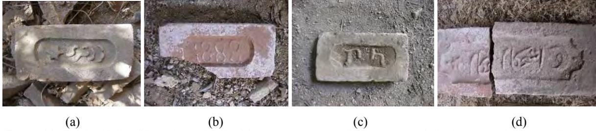
Figure 11: Bricks (6x10x23 cm.) used in building components of Edirne Ayvazbaba bastion (a) “Dimitri” script on the brick (b) “1888” dated brick (c) symbols on the brick, 2011, (d) “fortification” script on the brick Aynalibag Bastion, 2011.
