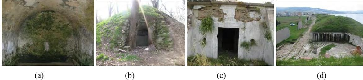
Figure 12: (a) Interior walls covered with moss of powder magazine of Kumkale Bastion, 2013, b) Vegetation problems in entrance of powder magazine of Bosna Bastion, 2013, (c) Vegetation problems on the exterior walls and plasters of powder magazine of Bolayir Merkez Bastion, 2013.
