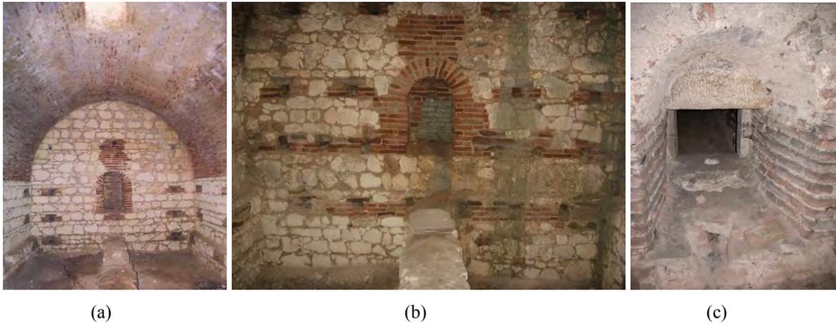
Figure 10: brick stove nich, ventilation holes and vault of garrison of Kırklareli Seyfioglu bastion, 2005 (b) brick horizontal beams, stove niche and ventilation holes of Garrison of Kırklareli Tas bastion, 2009 (c) A detail of ventilation shaft of garrison and quarter building of Hidirlik Bastion, 2009
