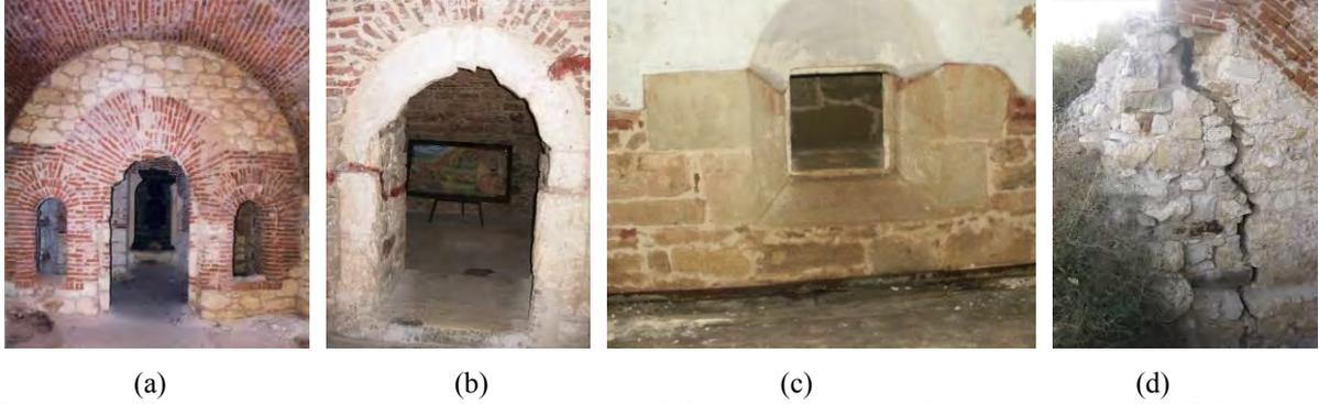
Figure 9: (a) brick door and windows arches and vault of Garrison building of Seyfioglu bastion, 2005 (b) coarse sandstone passageway wall of garrison and quarter building of Dortkaya bastion, 2013 (c) ashlar window of ordnance depot of Namazgâh Bastion, 2013, (d) segregated, rubble stone retaining of walls powder magazine of Aynalibag Bastions, 2011.
