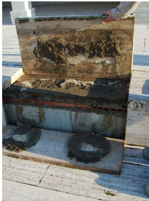
7-8. The removal of the travertine slabs on the bleachers of the *cavea* (left), and a particular of the poor sealing between the slabs and concrete structure of the parterre (right), photo 2013.
