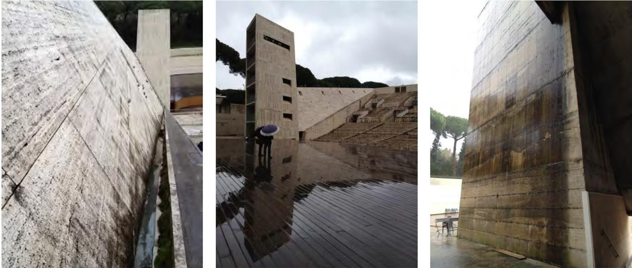
4-5-6. Degradation of the travertine slabs on the side prospects of the *cavea* (left), of the wooden plank of the stage (center) and of the concrete surface of the stage towers (right), photo 2013.
