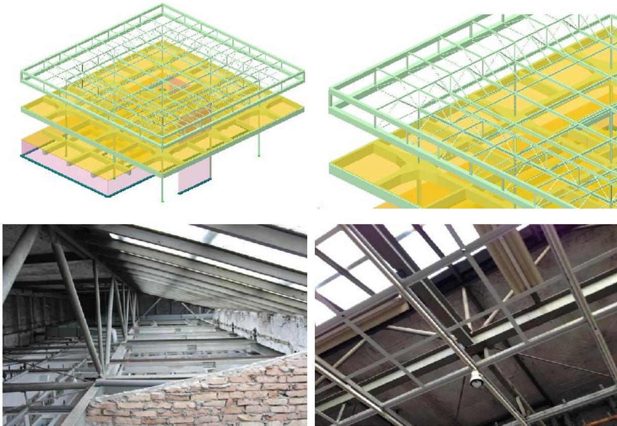
Figure 7: Tower 7 - 3D model of the steel structure and existing condition of the roof structure
