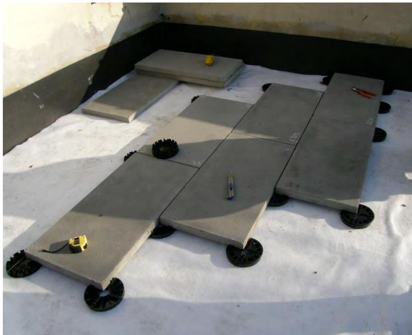
Figure 5: Multifamily house (former building for childless couples and single people) designed by Hans Scharoun, WuWA model Werkbund estate built in Wroclaw (former Breslau) in 1929. Roof recreation terrace of left wing during the last renovation - pavement slabs 40 x 80 cm, 4 cm thick (reinforced concrete). Phot. J.Urbanik, 2013.
