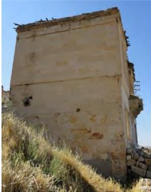
Figure 11, Tie bars on the wall (Ürgüp, block/lot: 131/45)
