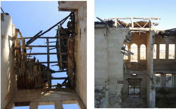
Figure 23-24, Intermediate stringer, Timber roof (Ürgüp, block/lot: 131/45)
