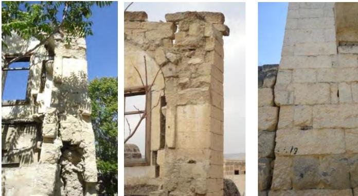
Fig. 9, Timber tie beams on the wall (Mustafapaşa, block/lot: 73/5112-B)
