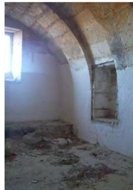
Figure 15-16-17, Vaults (rib arches and cover arches) (Ürgüp, block/lot: 182/10) (İ. paşa, no: 26b) (Ürgüp, block/lot: 131/23)
