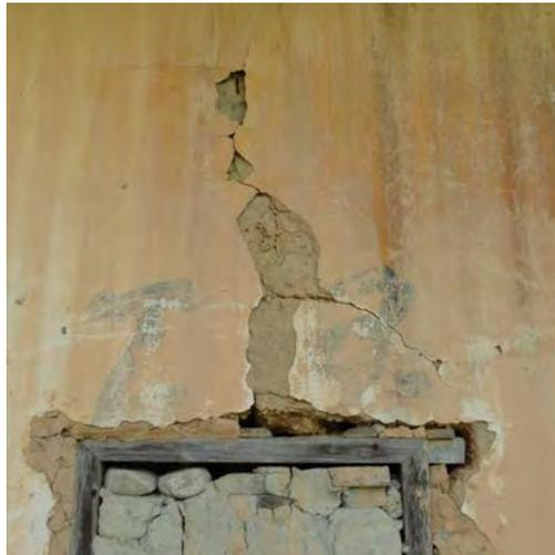
Figure 5: Cracks within hammed earth wall caused by subsequent window opening
