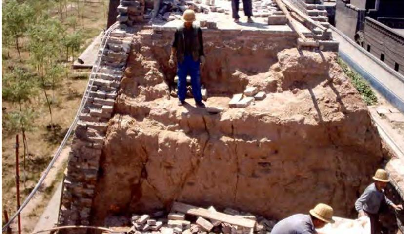
Figure 4: Complicated crack system within the city wall of Pingyao
