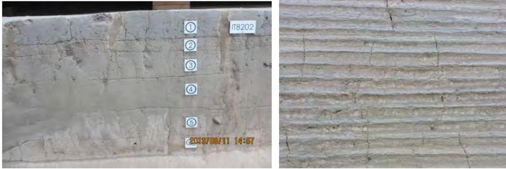
Figure 2: Cracks due to shrinkage
