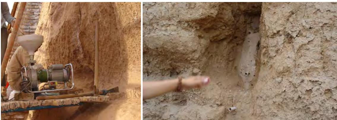
Figure 8: Voids filling with lime earth mix (photo by Li, Y. , personal information)
