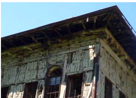
Figure 27: Timber frame, adobe filling
