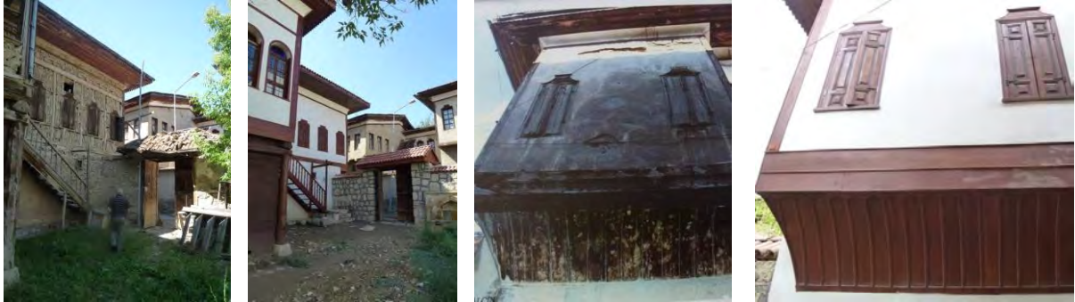
Figures 33-36: Northern and western (street) facades, before restoration and after restoration.
