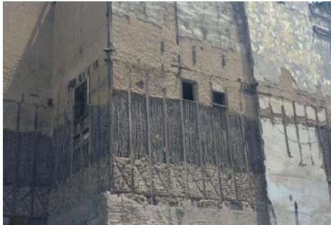
Figure 1: Exposed quincha on a building in central Lima
