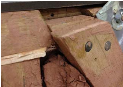
Figure 21: Failure of diagonal connection in test B3
