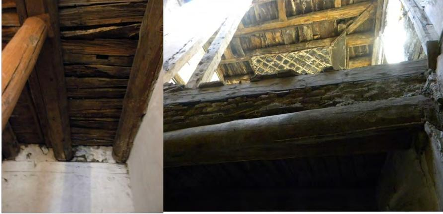
Figure 8: The section of mezzanine floor, it is composed of wooden beams and bricks (İnan, 2010)
