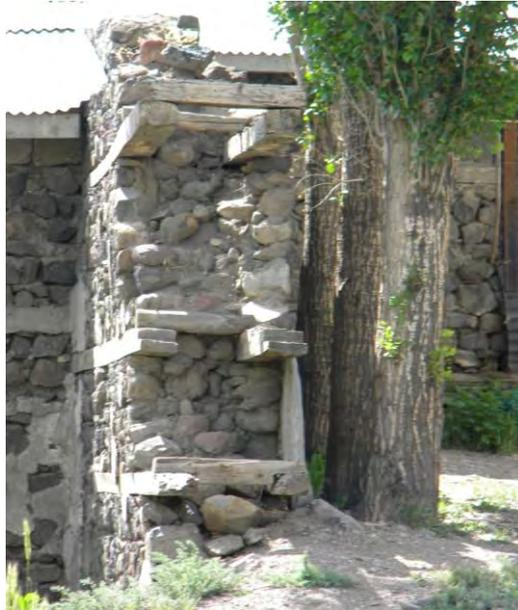
Figure 6: The runner beams at the wall (İnan, 2010)
