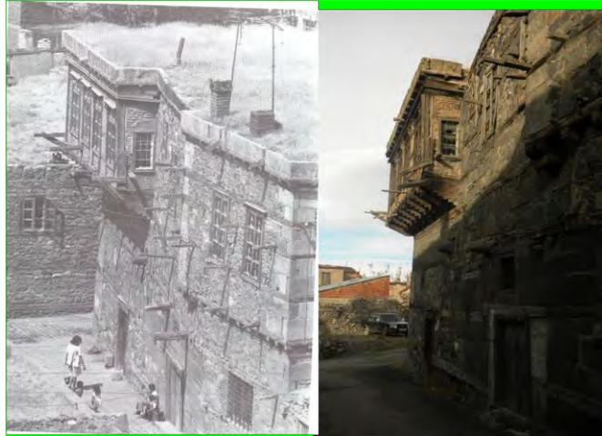
Figure 10: Only for Erzurum as a peculiar feature, püştüvan was extended approx. 50-70 cm. from out edge of the wall. It is used as scaffold during maintenance
