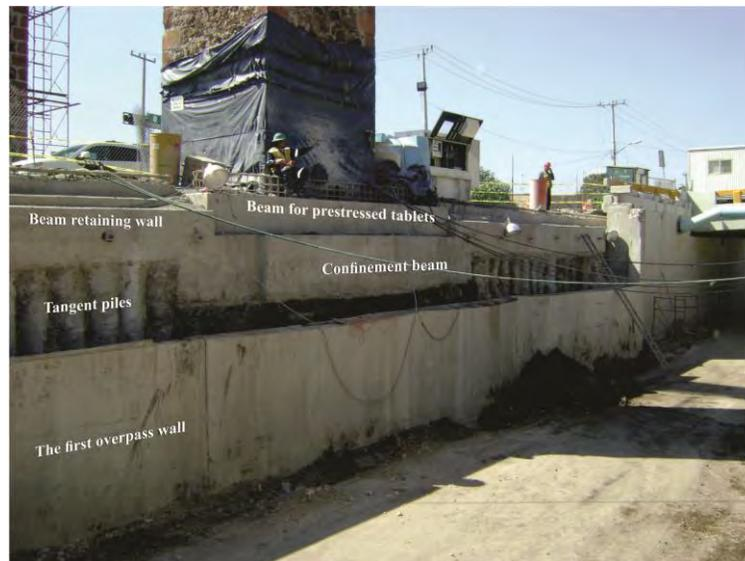
Figure 6 Overview of the beams
