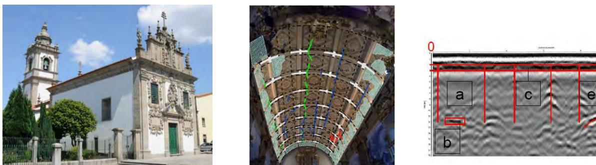
Figure 6 – Details of the St. Vincent Church in Braga - elevation (left); damage and deterioration in the main vault (center); GPR inspection (right).
