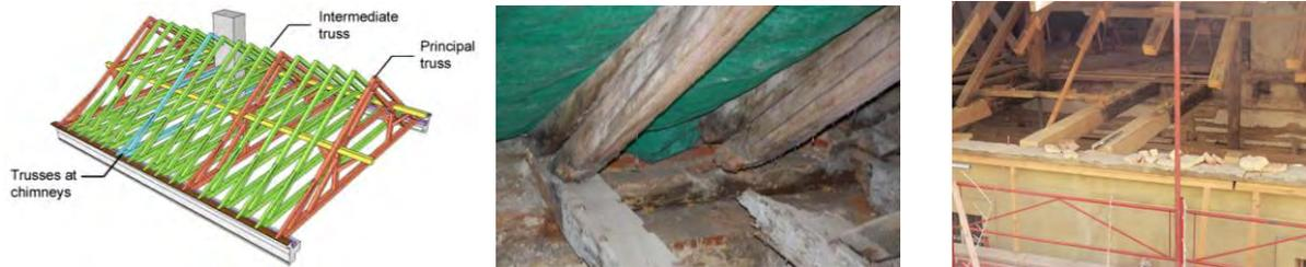
Figure 5 – Schematic of existing roof system (left); rotted ends of trusses (center); timber repairs during restoration (right)
