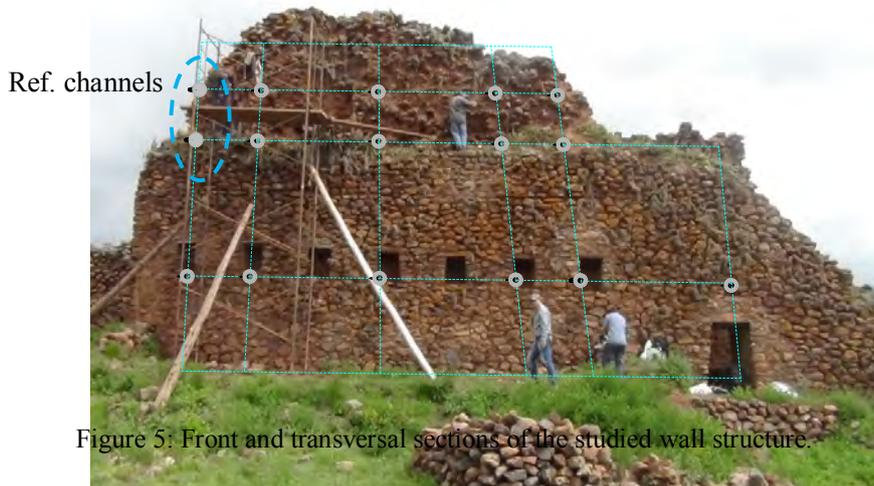
Figure 5: Front and transversal sections of the studied wall structure.
