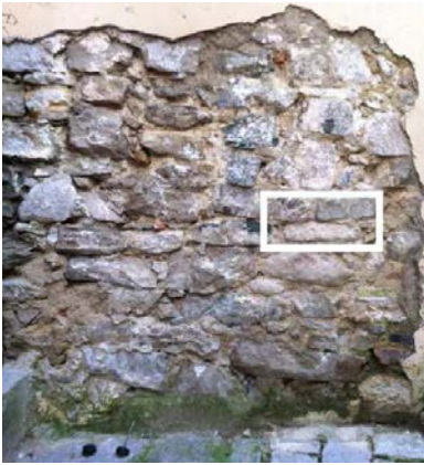
Figure 8: Residential building, Avigliano, panel B.
