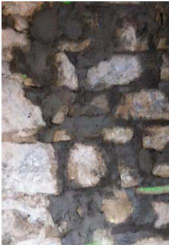
Figure 3: Joint repointing with new mortar.
