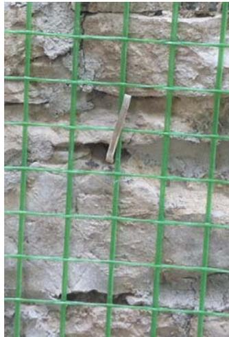
Figure 4: Application of the GFRP grid and anchors.
