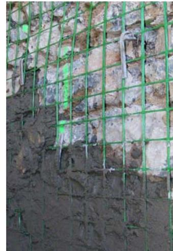
Figure 5: Application of second layer of mortar.
