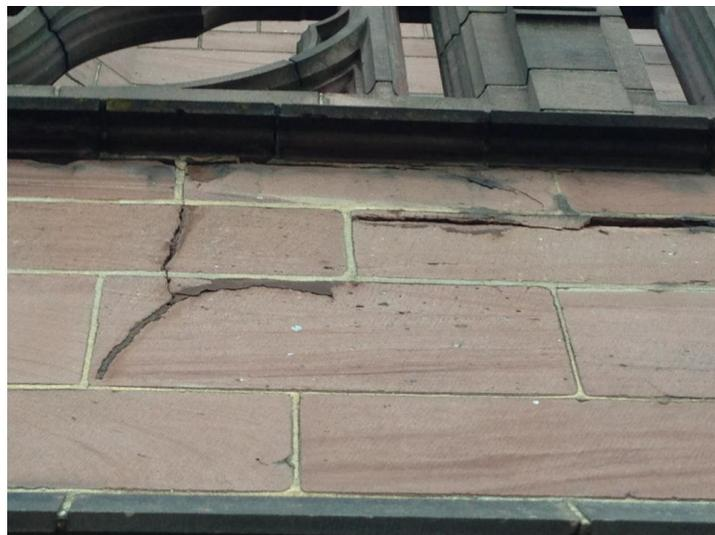
Figure 4: Inappropriate repair on outer surface of the Liverpool Anglican Cathedral has caused further crack and damage.
