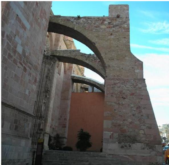
Figure 3: Buttresses in the north wall.
