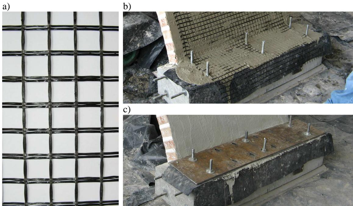
Figure 2: a) Glass fiber grid used in the study – detail. b) Glass fiber grid arrangement above the abutment – during application of the strengthening – vault VG-An. c) View of the strengthening's anchorage on the abutment of vault VG-An.
