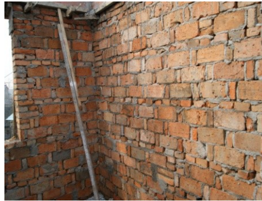
(b) In-Situ picture of rowlock cavity walls
