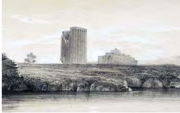
Figure 2: Historical painting of the damaged tower (1840s) [2]
