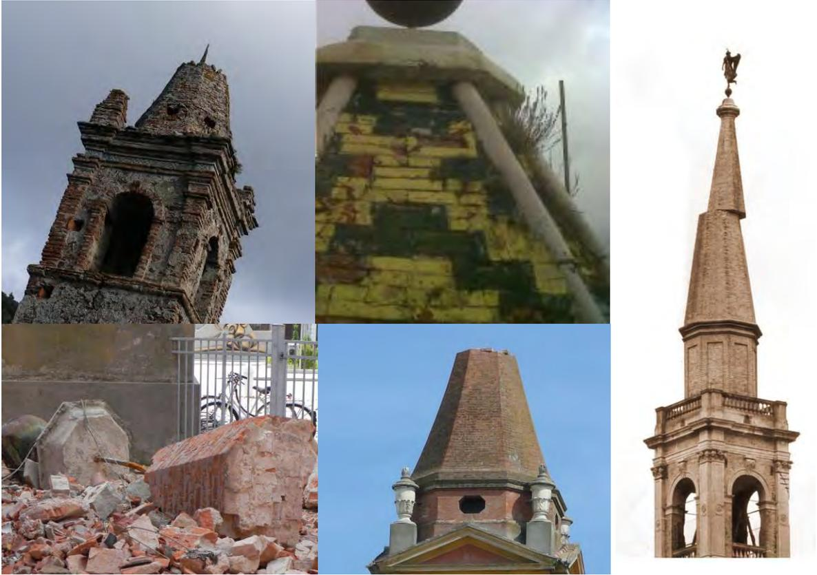
Figure 2: Some examples of seismic collapses of spires in different areas and at different levels. From top left, clockwise: Madonna dell'Alica di Pietrapennata (Calabria), Campobasso (Molise), Cordenons (Friuli - photo by Gigi Cozzarin), Sant'Agostino (Emilia), with the detail of the collapsed top element.
