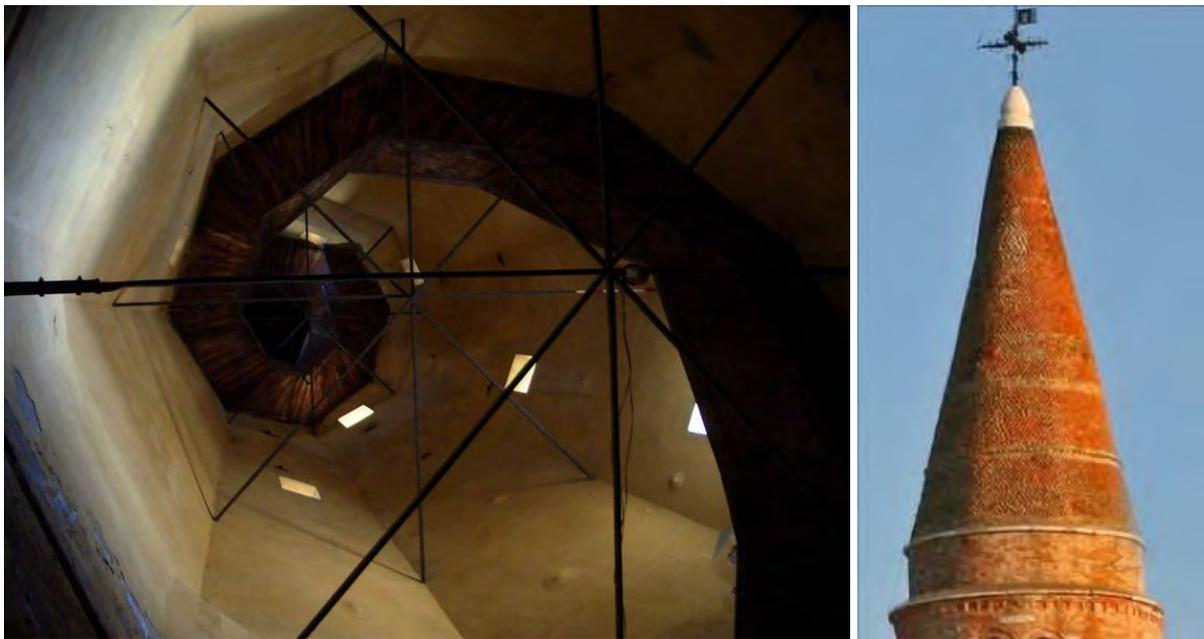
Figure 1: Traditional strengthening techniques for masonry spires: radial tie rods in the Ghirlandina tower in Modena (left), iron rings in the Caorle Cathedral (right).
