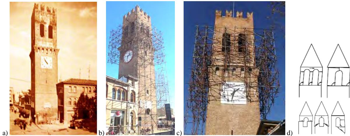
Figure 4: Civic Tower of Suzzara (a). The damage mechanism seems caused by the rotation of the corner pillars and by the following corner expulsion (b-d)
