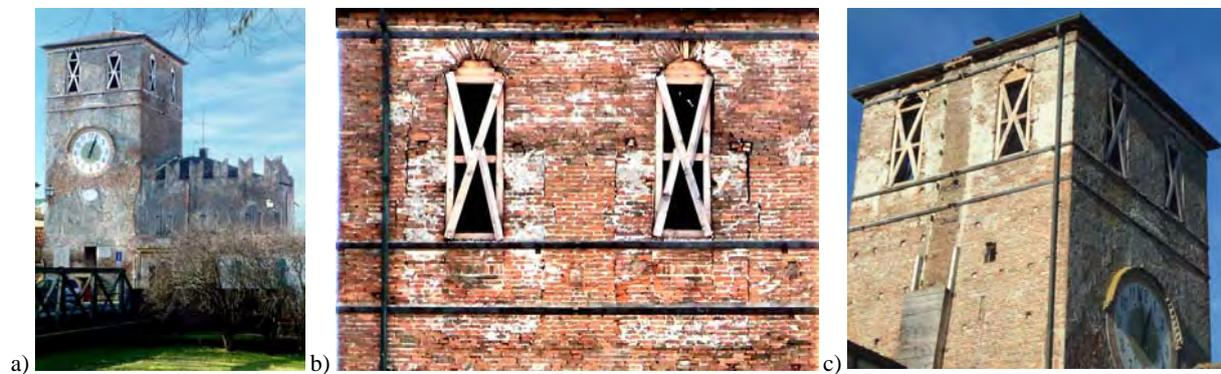
Figure 9: Torre Matildica a Bagnolo San Vito (a). The presence of several discontinuities in the upper area (b) of all the fronts was due to the constructive phases not effectively linked is evident from the cracks at the interface, and reinforced by both local supporting wooden frames both tie-rods elements to tie the top of the tower (c).
