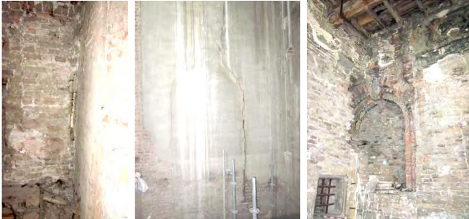
Figure 12: Palazzo del Podestà in Mantua. Examples of damage related to the lack of effective connection between the historic building phases.
