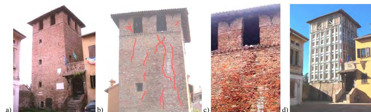
Figure 7: Tower of Prisons at Gonzaga before the earthquake (a); the formation of deep vertical cracks (b) in the south side was caused by the overturning mechanism of the south-west corner (c), and highlighted by an apparent out of plumb which justified the massive emergency intervention for the safety of the tower itself (d).
