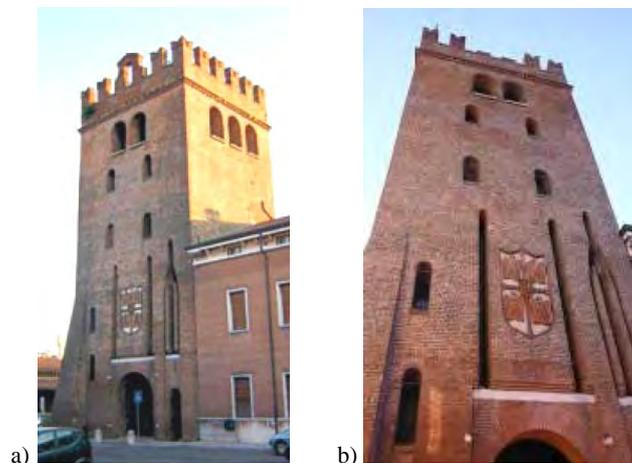
Figure 3: Civic Tower of Sermide before (a) and after the earthquake (b). The reported damages included the partial collapse or damage to the battlements.
