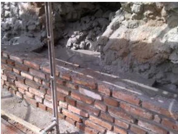
Figure 8: Infilling masonry in collapsed wall.
