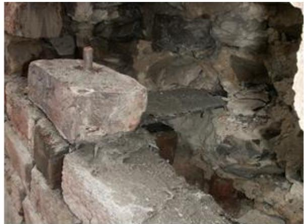
Figure 13: Elements joining together external leaves – an anchor.
