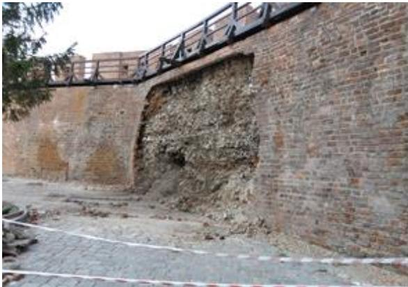
Figure 3: Eastern part of the wall and its damaged 8 m long section.
