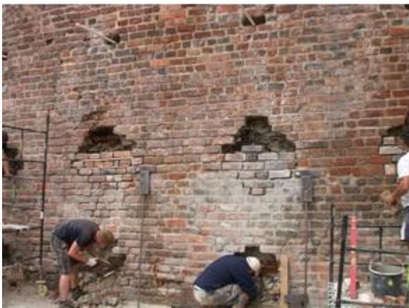
Figure 12: Elements joining together external leaves – anchor arrangement.
