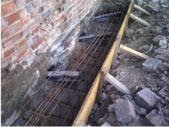
Figure 10: Pile cap reinforcement.
