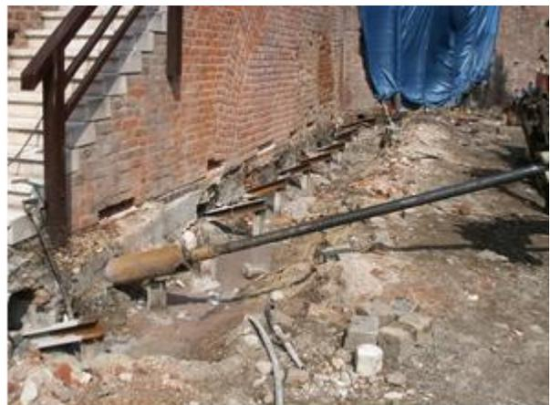
Figure 9: Drilling of holes and installing pile cantilevers.
