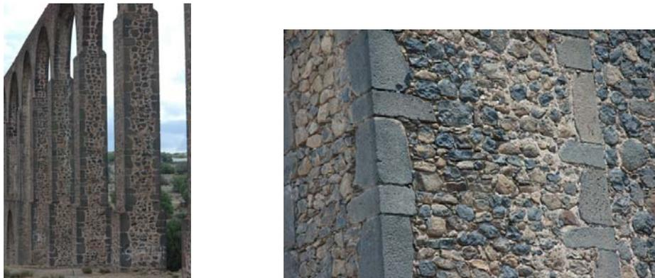
Figure 3: Arrangement of stone masonry in columns.
