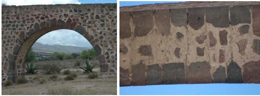
Figure 4: Arrangement of stone masonry in arches (view from the side and view from the intrados).
