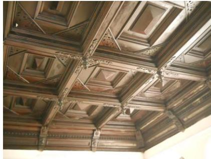
Figure 5: Coffered ceiling
